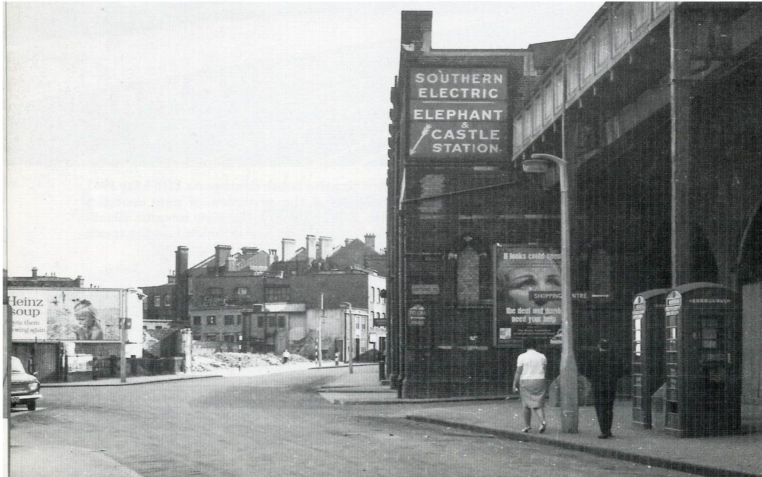
Note the tall steel platform supports on the right from the 1925 campaign extending the station's platforms.
