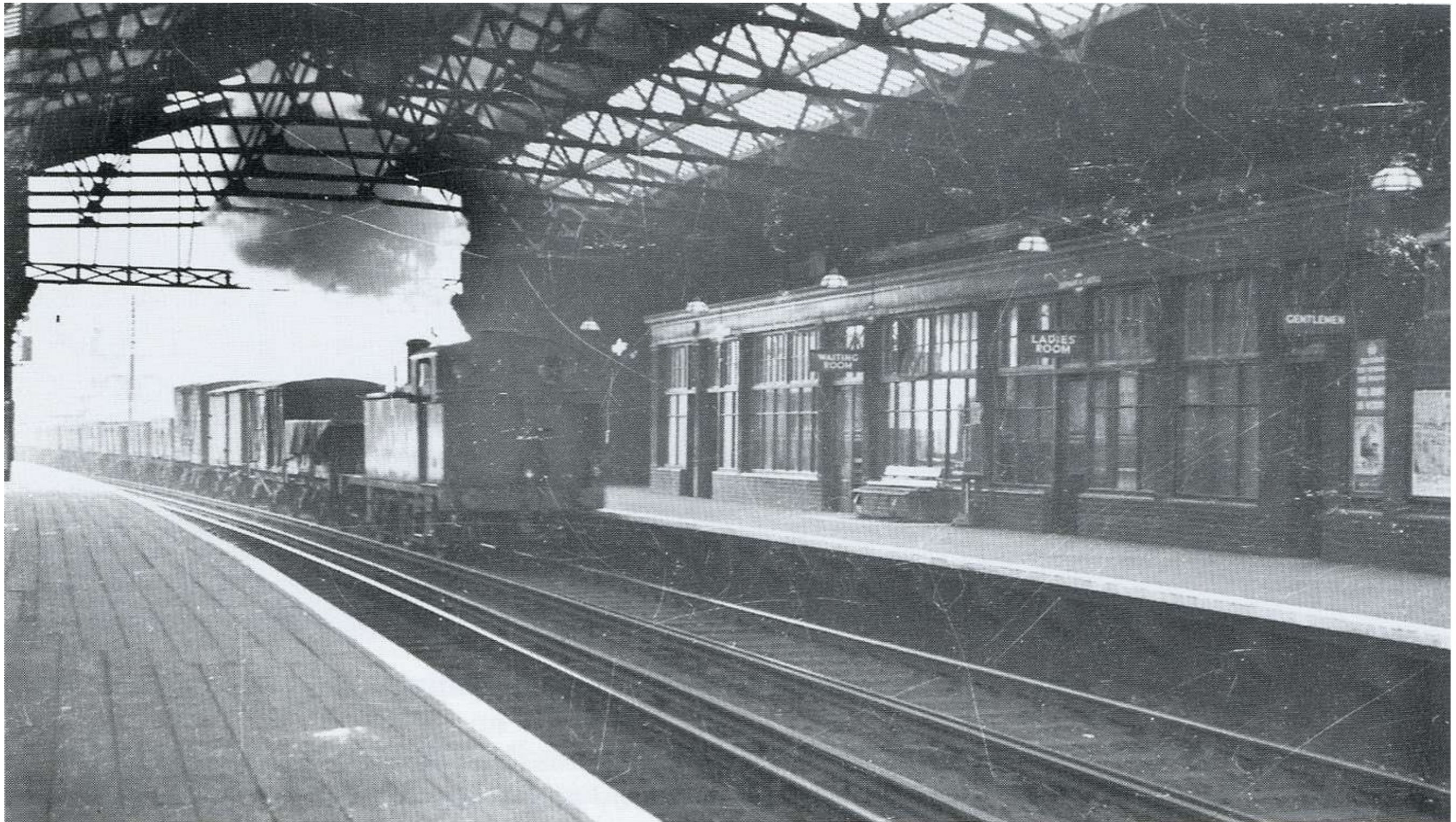
This fascinating photo shows what is probably the original Victorian railway roof. This could offer some clues to enhancements for the platform 1 elevation (see page 12 for roof exterior view).
