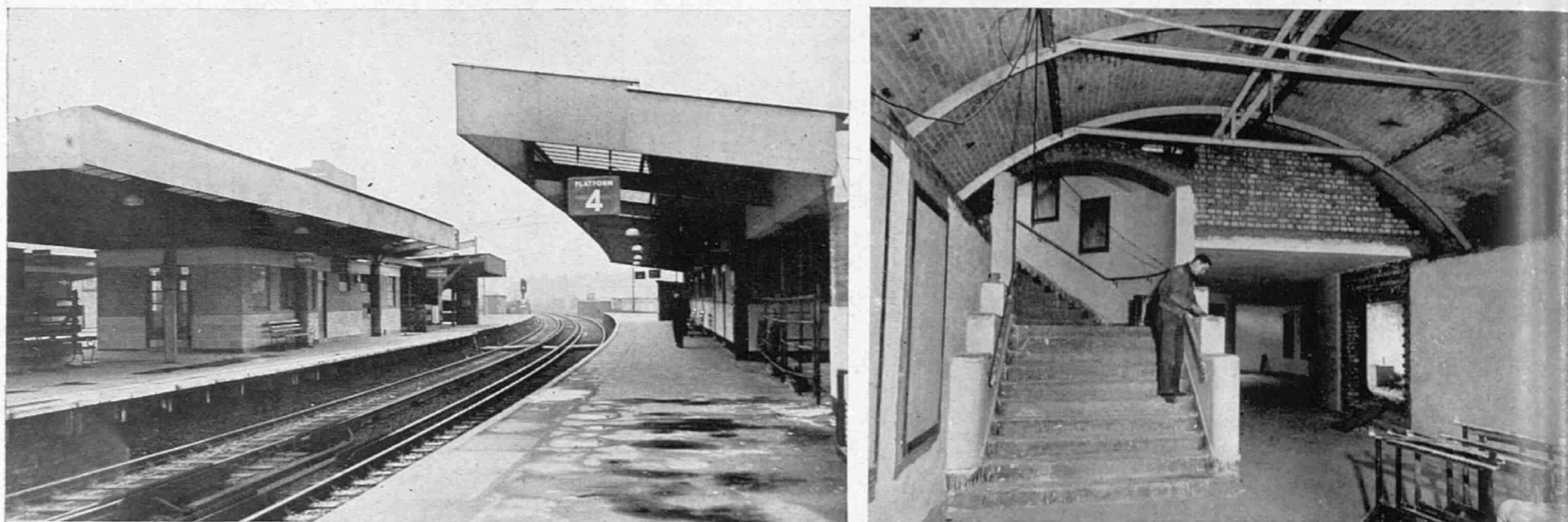
THE PREFAB STATION : THE REBUILT ELEPHANT AND CASTLE STATION, ON THE SOUTHERN REGION : Left —The main platforms and the waiting rooms, where prefabricated materials have been largely used to rebuild the bomb-damaged platform. Right —The entrance hall, in which pre-cast concrete has been employed
