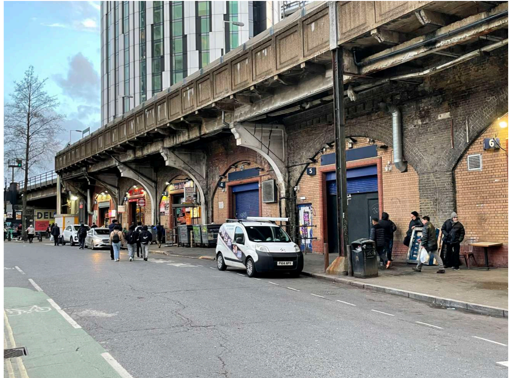
Present day view of the 1925 platform extension along Elephant Road, showing the cast in-situ ferro-concrete brackets and 'Main South-Eastern Line' platform on the East side of the station.
