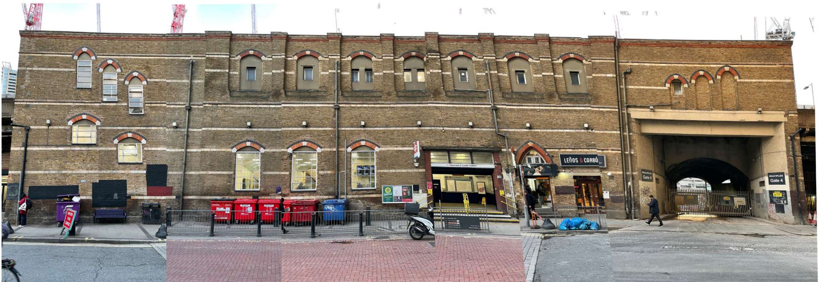
The current Elephant Road station facade. The main station was built in 1862 by the London, Chatham and Dover Railway Company. The station was extended and some of the interior remodelled in the 1920s by the office of the chief architect of the Southern Railway, James Robb Scott (1882-1965) following a fire, and repaired and reconstructed in the late 1940s/early 1950s after heavy bombing along the railway line during the Blitz (1940-41).
